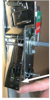
3. Adjust the lock support plate to be perfectly vertical on the door and temporarily secure it with a clamp. During this operation, check the proper functioning of the latch and lock (auxiliary latch) spindles. The lock spindle should extend backward, bypassing the repetition lock.
