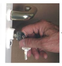
1. Remove the casing (turn the cylinder key to the left).
