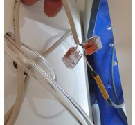
Connect the bare electrical wires to the cable with WAGO connectors, passing through the central hole at the back of the panel
