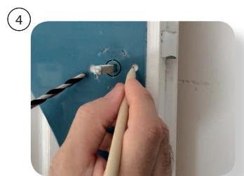
To show red side of plate (adhesive) in the square spindle, to identify the holes on both sides of this square spindle, then to carry out drilling in Ø6 mm if your lock presents the same spacing of holes envisaged for this purpose in order to allow the installation of the relay screws.
