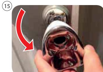
It is now possible to install the ul-101 handles by clipping them on their mechanisms, unless one has to carry out the consistent optional adjustment by adjusting one of the 9 handle positions.
