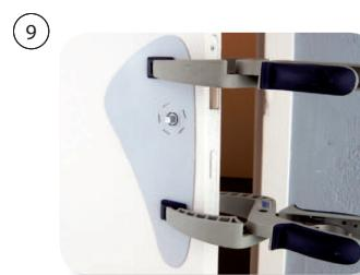
To fix the plate on the door using grips, during at least 30 minutes, in order to optimize its adherence then, once the grips removed, to withdraw protection film.
