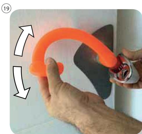
To clip the UL-101 handle on "the nut with the 3 red O rings". To check its height. If it is suitable, congratulations your UL-101 system is ready to be used.
