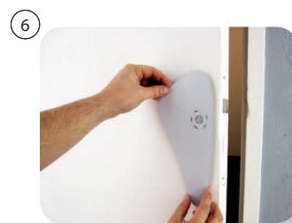
To stick the finger-plate on the door by using the square spindle as an installation template.
