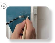
To show red side of plate (adhesive) in the square spindle, to identify the holes on both sides of this square spindle, then to carry out drilling in  $\emptyset 6 \text{ mm}$ if your lock presents the same spacing of holes envisaged for this purpose in order to allow the installation of the relay screws.
