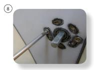
To install the 2 relay screws (if your lock allows the boring of holes).
