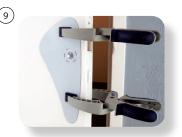
To fix the plate on the door using grips, during at least 30 minutes, in order to optimize its adherence then, once the grips removed, to withdraw protection film.
